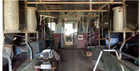
Before: Dairy facilities unused for 15+ years
