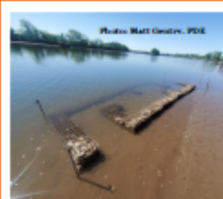
Figure 1: Recycled oyster shell gabbions to help restore freshwater mussel beds at Bartram's Garden along the Schuylkill River in Philadelphia, PA.
